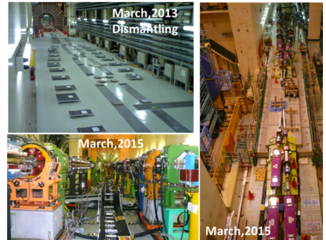
Figure 4: The beam line of \sim 320 m around IR has been reconstructed completely.
