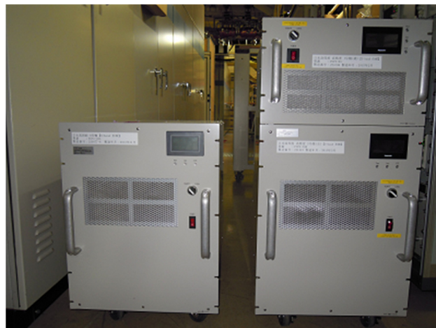
Figure 1: Outward appearances of the normal model (left) and highly precise model (right) of Nikoha CCPSs [11].
