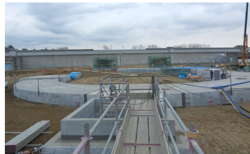
Figure 7: DR tunnel under construction.
