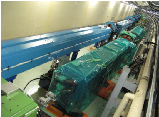
Figure 2: New 4m bending magnets for the LER.
