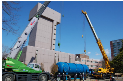
Figure 3: Installation operation of the accelerator tank on the support.
