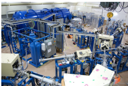
Figure 7: Panoramic photograph of the accelerator room (August, 2014).
