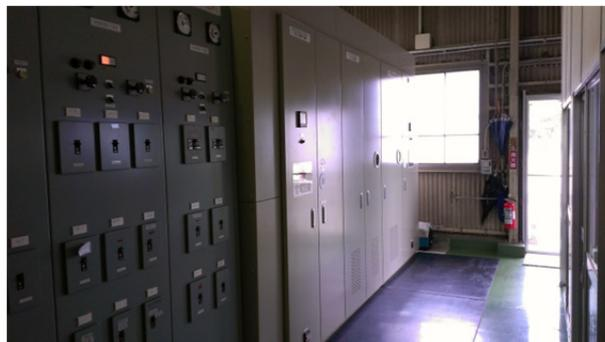
Figure 9: Relocated transformers for klystron modulators and cooling systems from the radiation controlled area.
