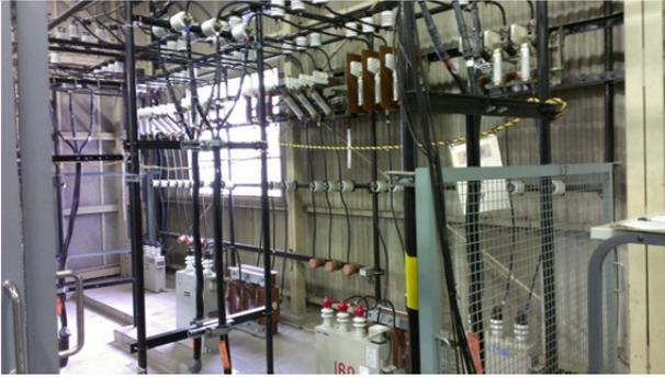
Figure 10: Newly built automatic power factor regulator.
