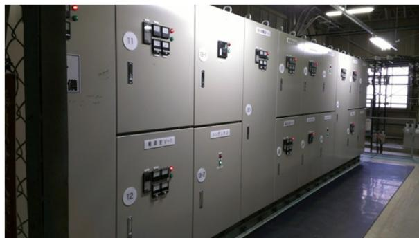
Figure 8: Renewed relays and circuit breakers.
