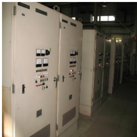
Figure 5: Oldest quadrupole powers supplies in PF-AR.
