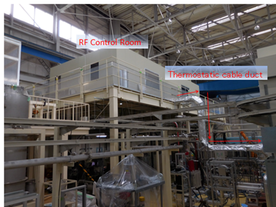
Figure 1: RF control room (outside view).
