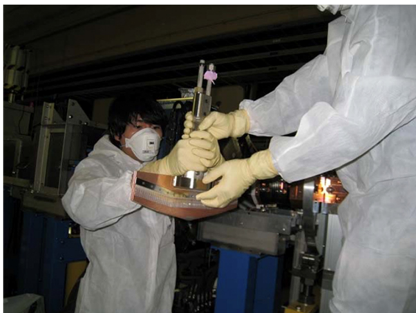
Figure 4: Replacement work of D02V1 collimator jaw.
