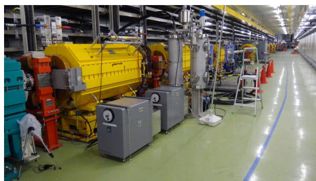
Figure 2: Cable connection devices and chemical filters.
