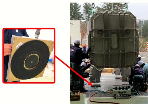
Figure 10: Setting of the air caster module.
