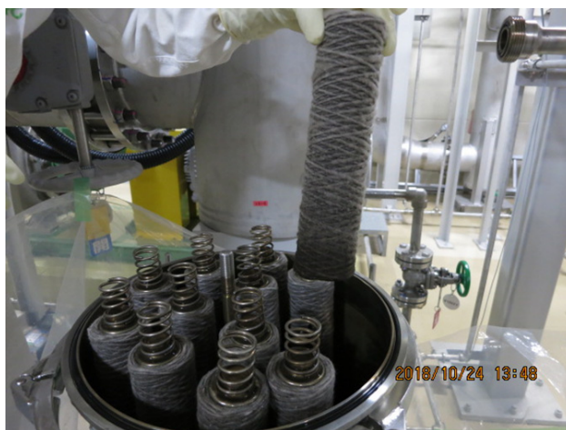
Figure 5: Replace a filter of RI4 water cooling system in J-PARC Linac.
