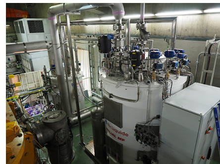
Figure 3: Cold box and joint box are installed in the linac building.
