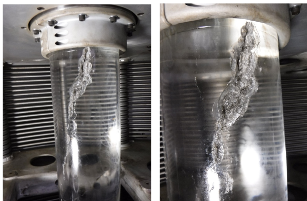
Figure 6: Rotating shaft cracked by electric discharge. Left is an enlarged version.
