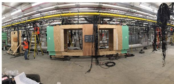
Figure 6: Wooden mockup of the  $\beta=0.085$  cryomodule to check mechanical interference and temporarily route cables for termination.
