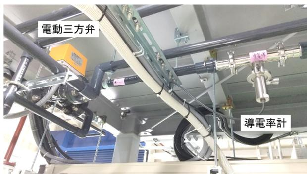
Figure 5: The electric 3-way valve and the conductivity meter.
