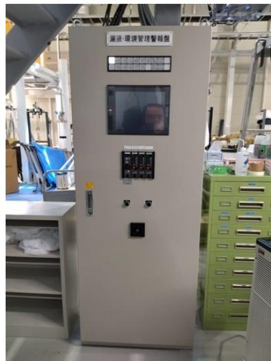
Figure 7: Environmental safety alarm panel to control each safety device.
