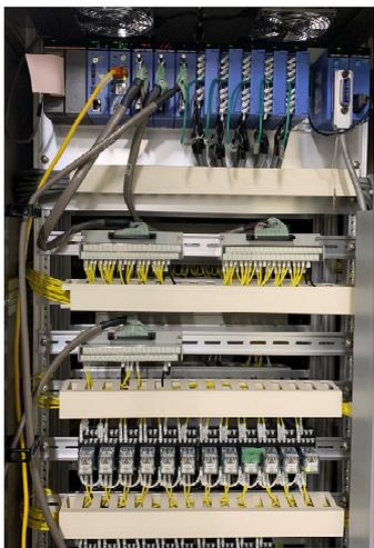
Figure 2: Yokogawa PLCs and relays for NEOMAFIOS and SC-ECR. Same system is also used for polarized ion source which is not shown this time.
