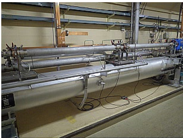
Figure 6: State of cable connection in the tunnel.
