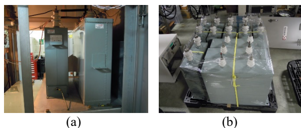
Figure 3: The removed smoothing capacitors. (a)The capacitors before removed in a modulator. (b)The ones after removed and stocked.
